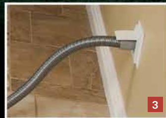
The vacuum inlets are strategically placed.
